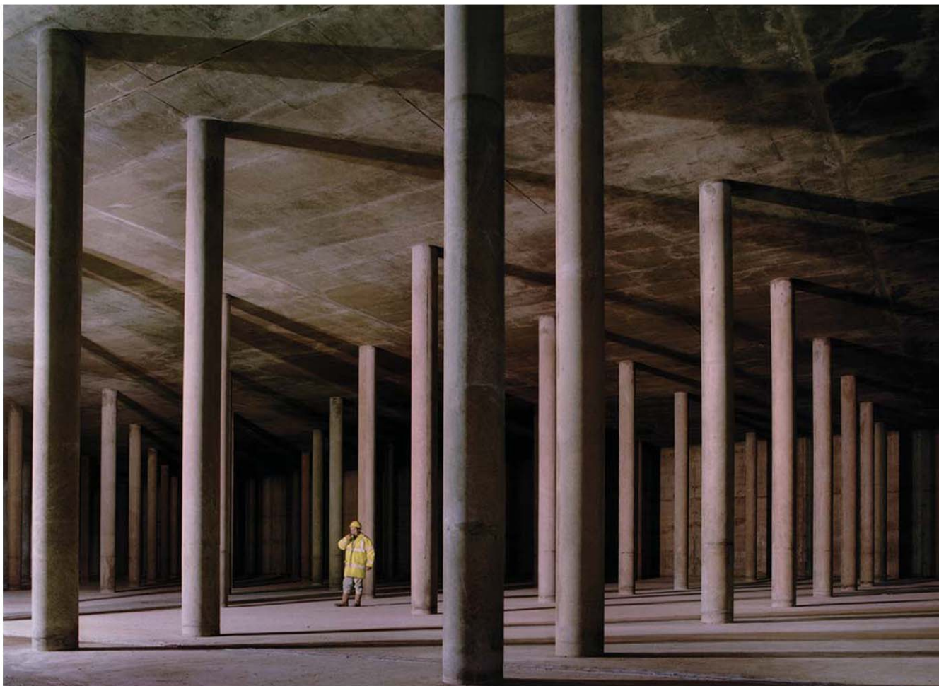
Bedford: New 45,000m 3 reservoir (courtesy Laing Construction)
