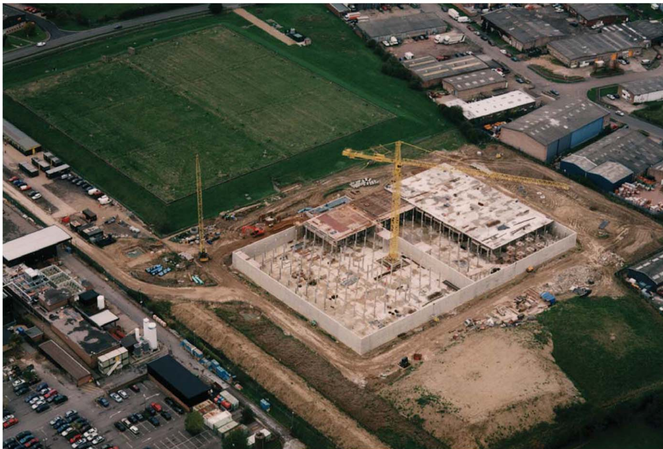
Bedford: Construction of new reservoir at Manton Lane (courtesy Laing Construction)
